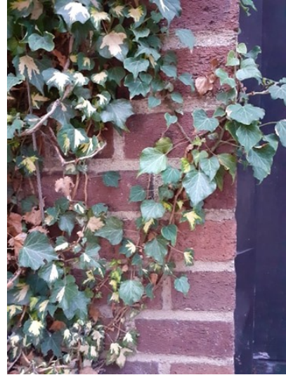
FIGURE 1.2: Ivy branching attached to a wall at Queens University Belfast (Personal collection)
